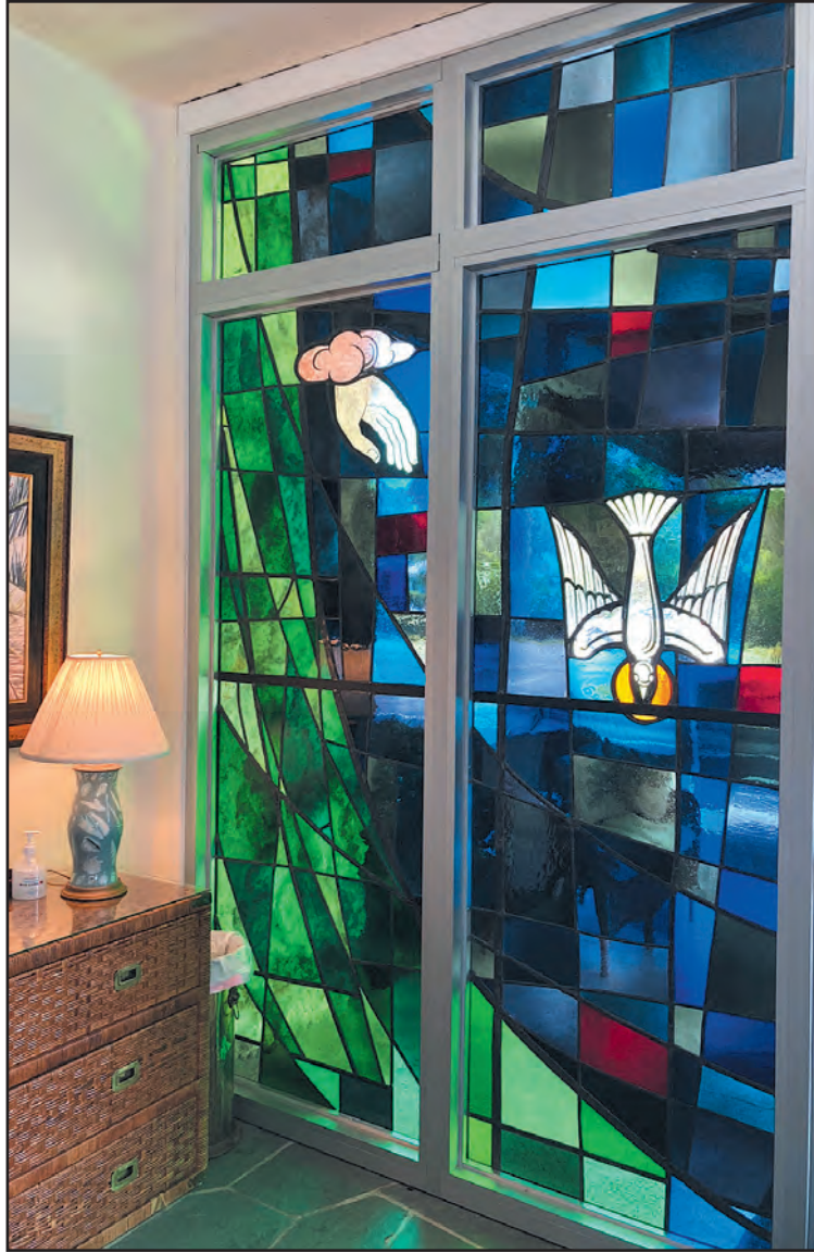
LEFT: Safely reinstalled behind impact glass, the panels in the narthex should be safe from hurricane damage. RIGHT: The stained glass windows and sweeping roof line help to define the interior of the church. Photos provided
