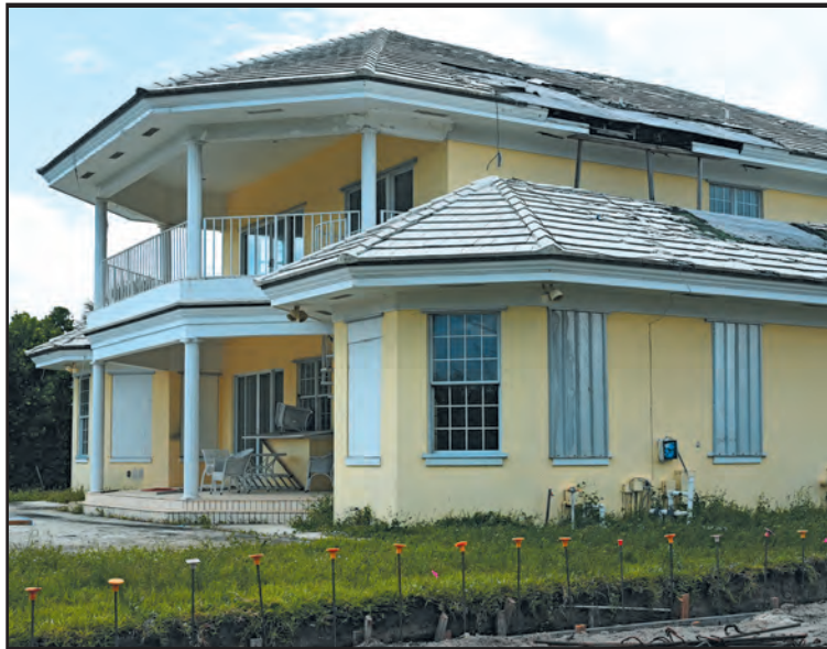
Temporary window coverings are just one of numerous problems for the house at 2900 Avenue Au Soleil, which the town hopes will be demolished. Jerry Lower/The Coastal Star
