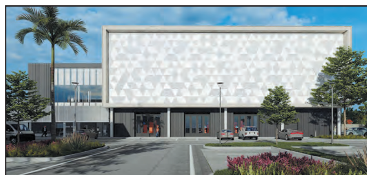
BELOW: The central energy plant, set to open in early 2024. Renderings provided
