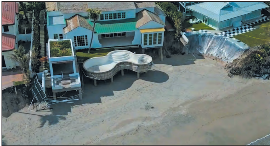
Jupiter Inlet Colony beachfront homeowners suffered damage this past winter during an unexpected weather event. Photo provided by WPEC
