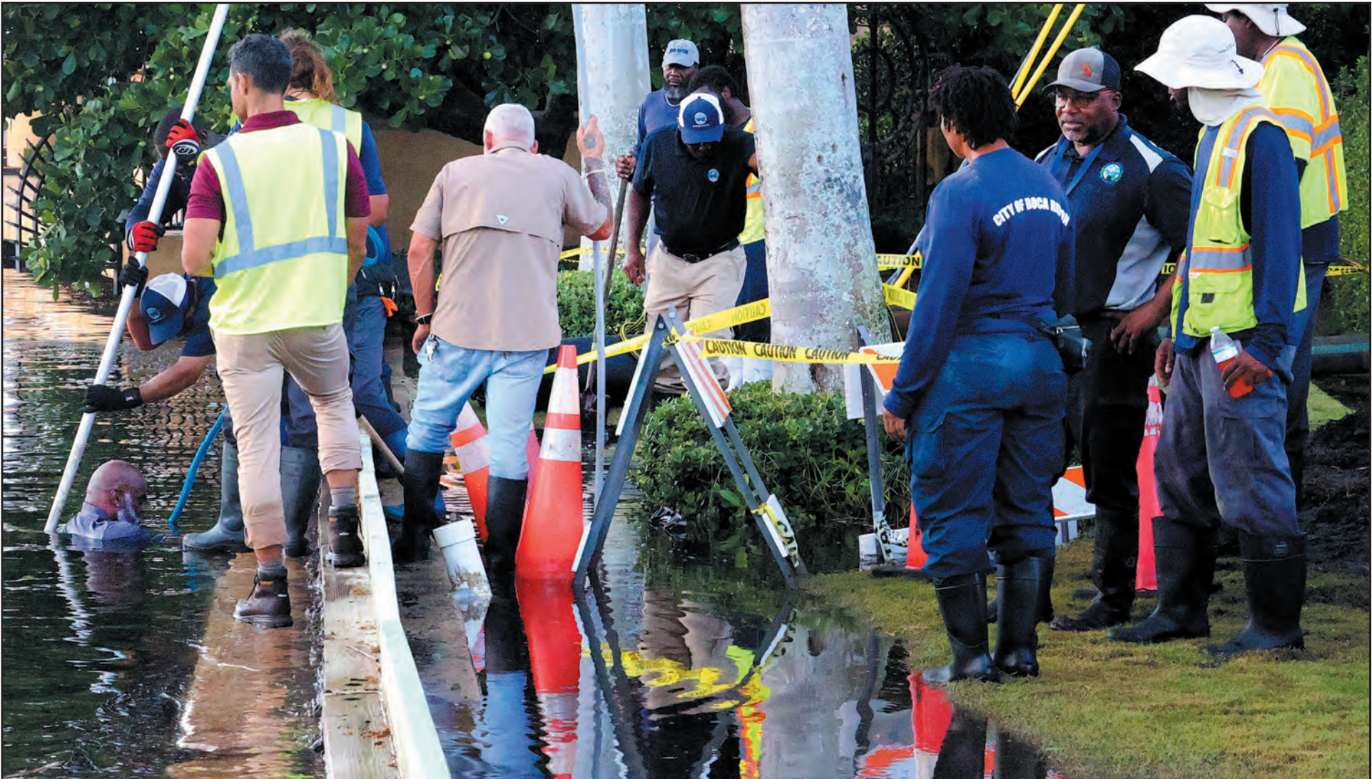
Eleven Boca Raton city employees assist Paul Baker, a stormwater supervisor, who was up to his chin fixing a portion of the sea wall cap along the south end of Wavecrest Way in the Por La Mar neighborhood on Oct. 9.
