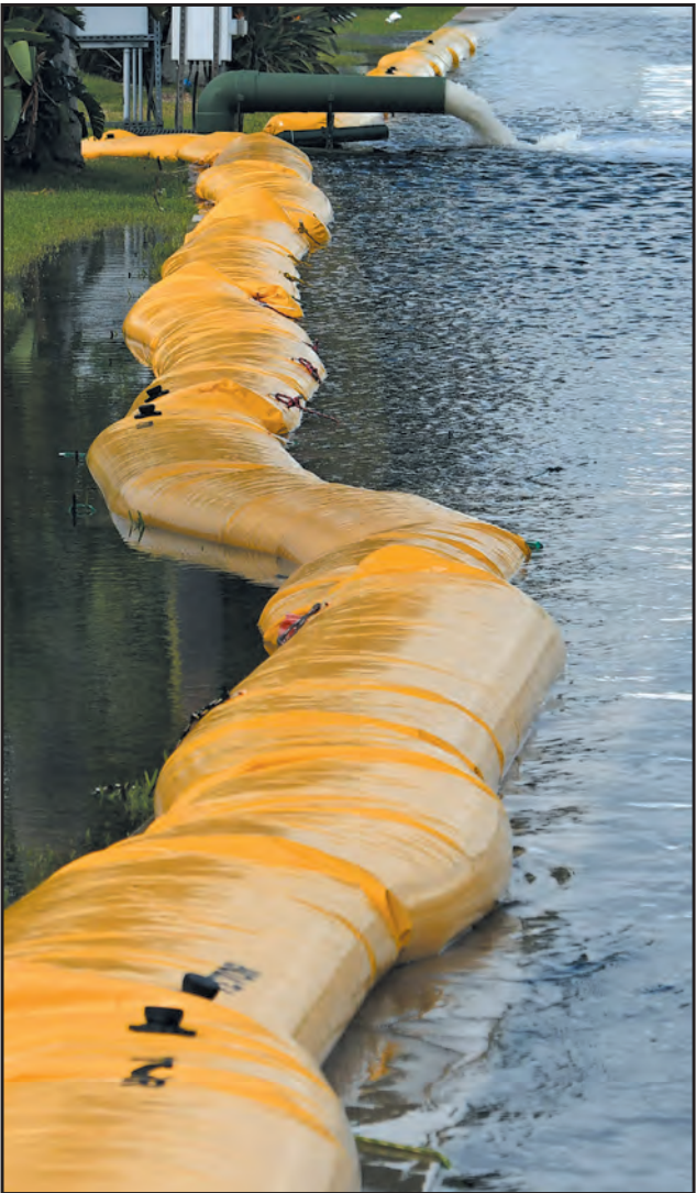
Some protective measures are helping to deal with typical king tide effects. LEFT: In Briny Breezes, water-filled plastic bladders sit atop the sea walls, and industrial size sump pumps in multiple locations on the west side of the community provide some protection from the king tides. ABOVE: The privately funded sea walls in Ocean Ridge near Anna Street did protect the homes of residents who paid for them, but could not protect the stairs down to the beach. Before October the sand at this location extended at least 5 feet beyond the concrete wall at high tide. Photos by Tim Stepien and Jerry Lower/The Coastal Star
