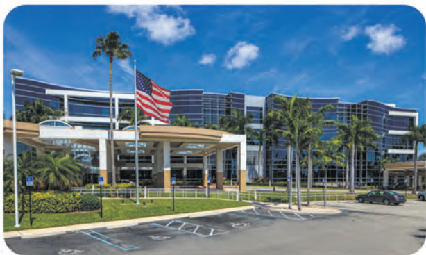
Bethesda Hospital East
