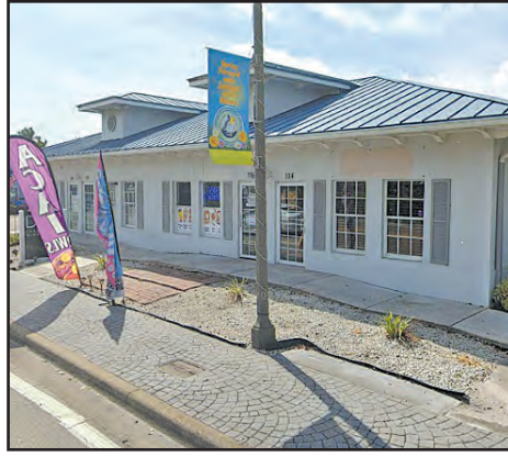
The owner of this retail center has been in a dispute with Lantana over code enforcement at the site.
