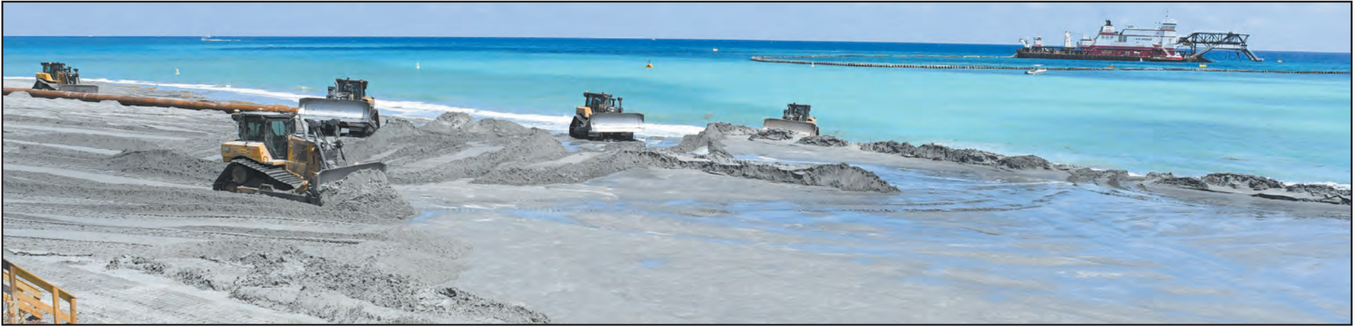
Five bulldozers level freshly pumped sand after it was spread onto the beach in Ocean Ridge from the dredge (at right) as part of a $9.4 million U.S. Army Corps of Engineers project. The gray color comes from organic sediment and is common for beach renourishment projects. It will change over time to the natural color of sand. The project is expected to continue through April, before the peak of sea turtle nesting season arrives. Jerry Lower/The Coastal Star
