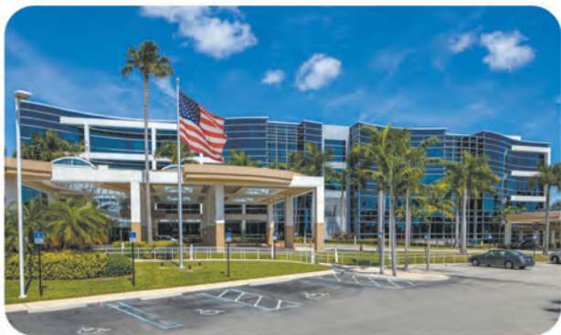
Bethesda Hospital East
