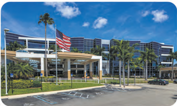
Bethesda Hospital East
