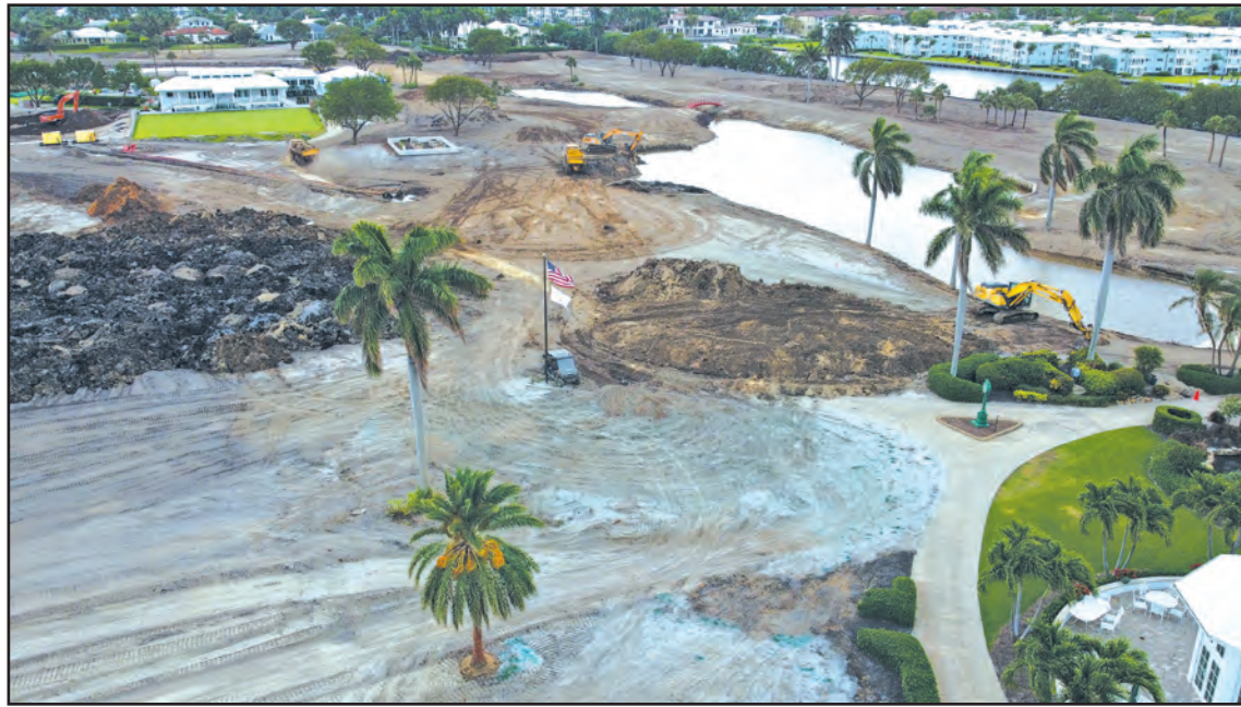
Bulldozers and backhoes work the grounds of The Little Club as part of the remake of the property. Jerry Lower/The Coastal Star
