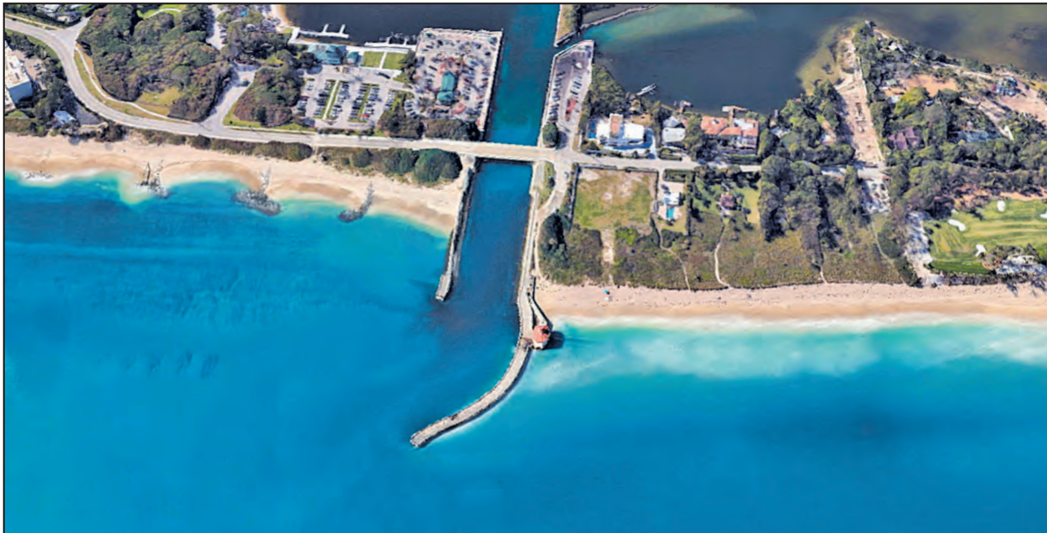
The sand transfer plant located on the north side of the Boynton Inlet pumps a slurry of sand and seawater through a pipe under the bridge, and onto the beach south (left) of the inlet. Photo provided by Google Maps
