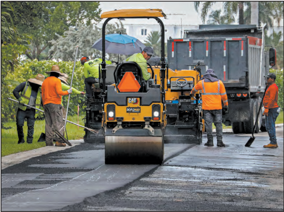
Workers lay asphalt in Gulf Stream’s Core area on July 27. The work is part of a two-year capital improvement plan. Tim Stepien/The Coastal Star
