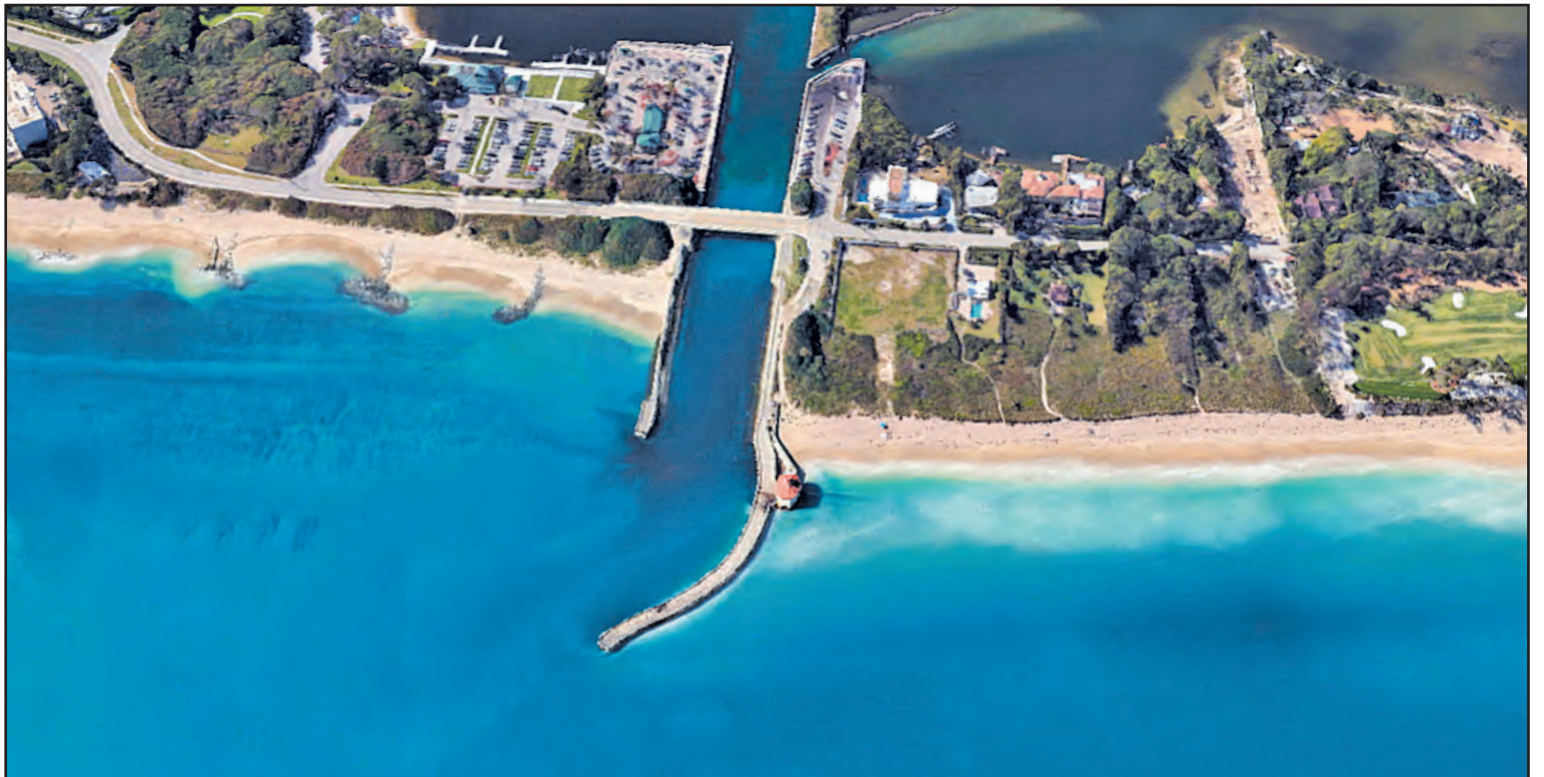
The sand transfer plant located on the north side of the Boynton Inlet pumps a slurry of sand and seawater through a pipe under the bridge, and onto the beach south (left) of the inlet. Photo provided by Google Maps
