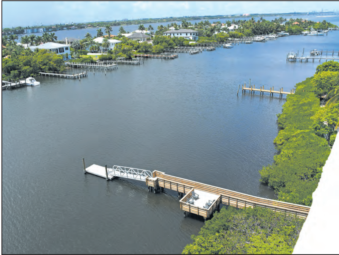
South Palm Beach says it has zoning control over docks like this one, seen from the roof of Concordia West. The wooden dock, which Lantana says should be demolished, has a floating kayak launch. Hypoluxo Island is visible across the channel. Jerry Lower/The Coastal Star
