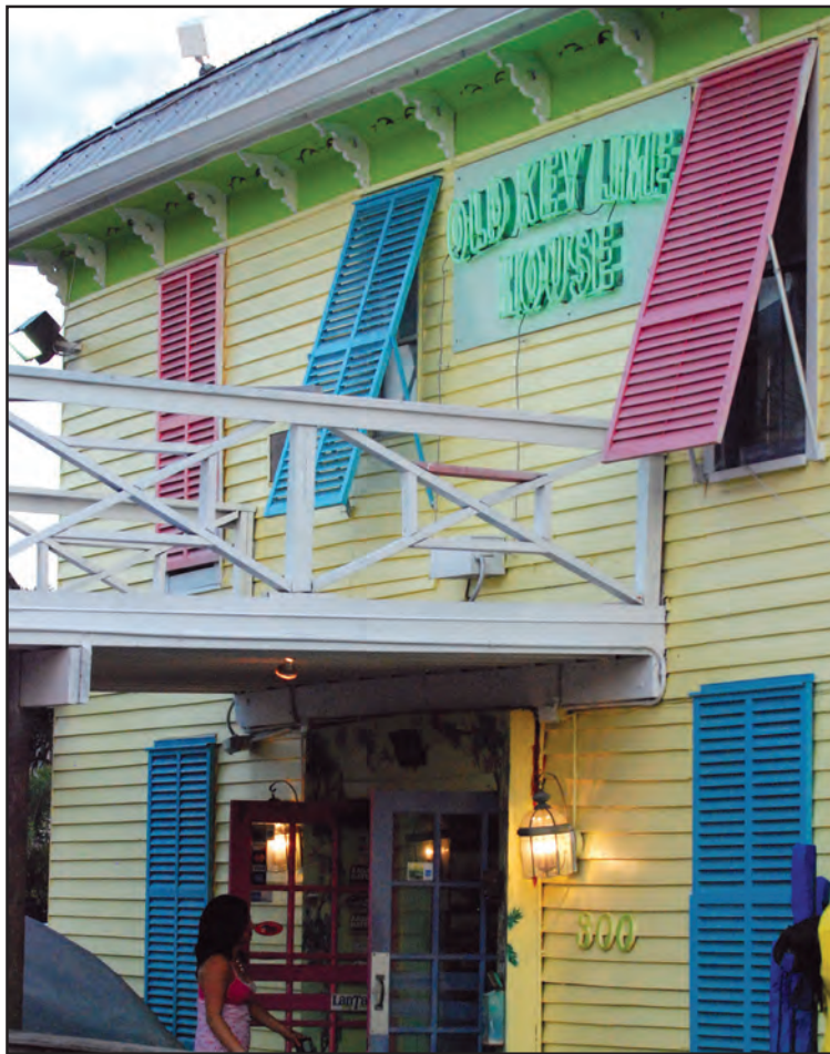
The steel Bahama shutters of Lantana's Old Key Lime House helped keep the 1889 building secure during storms. Photo by Jerry Lower
