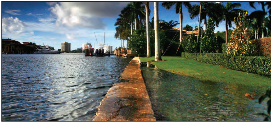
Lake Boca Raton crested over the sea wall and breached the Por La Mar neighborhood in Boca Raton. Photos by Tim Stepien/The Coastal Star
